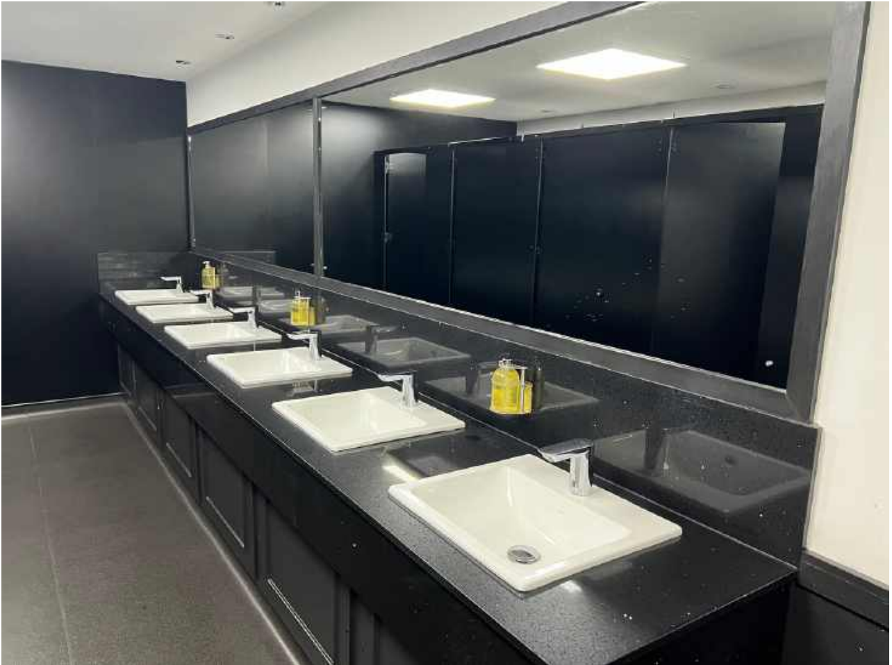
Image description: sinks in the upstairs female toilets.
