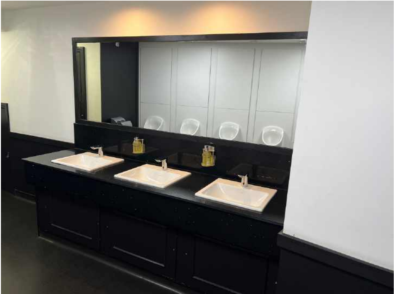
Image description: sinks in the upstairs male toilets.
